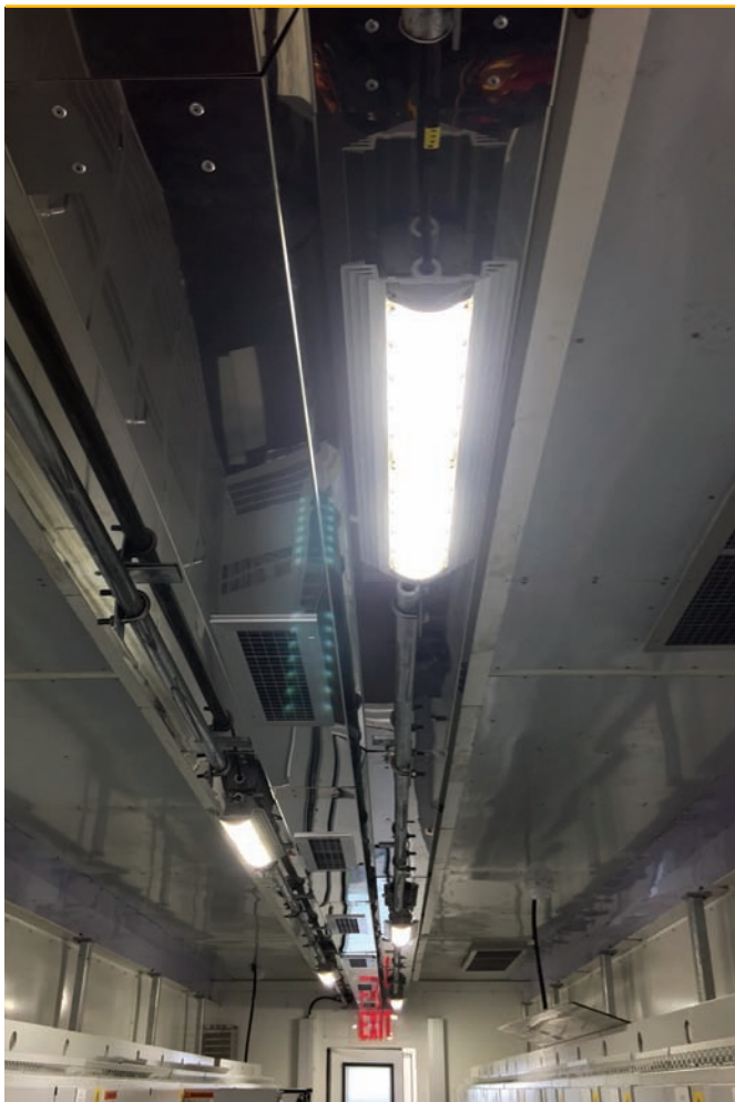
HDL2s in an electrical control room
