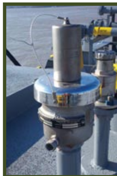
2.5" Equate PV Valve mounted on stand pipe next to 2" Sampling Ball Valve.
