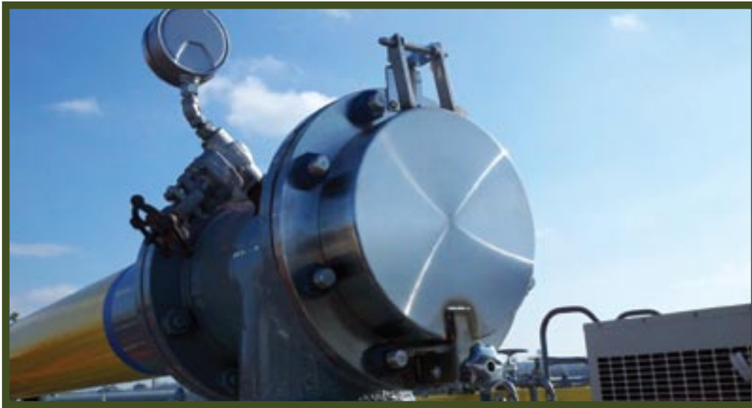
Typical Vapor Headers with ERL Vent Header Sight Glass and ERL Model 505 Pressure/Vacuum Gauge.
